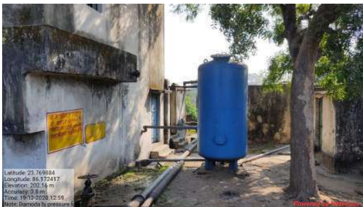
FILTER PLANT IN THE MINE AREA
