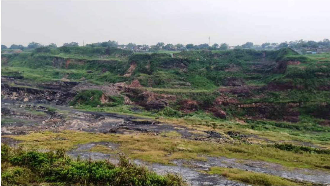
Figure 19: Subsidence area in Bagdigi Mines
